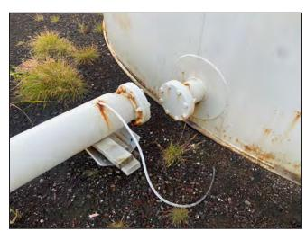
**Photo 28:** Overall view of bonding cable and blind flange (fuel transfer line)..
