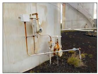
**Photo 16:** View of autogauge head, electronic gauging, and blind flange (fuel transfer valve).
