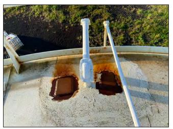
**Photo 36:** View of autogauge head and electronic gauging.
