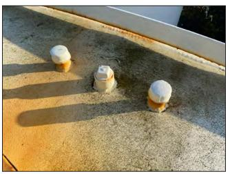
Photo 52: View of capped/plugged nipples.
