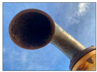
**Photo 38:** Detail view underneath gooseneck vent with no screen.
