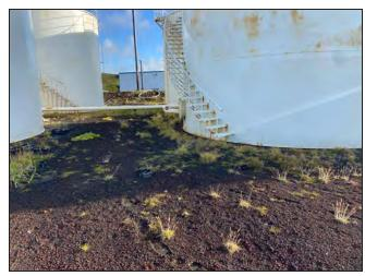
**Photo 58:** Overall view of tank foundation and earthen pad.
