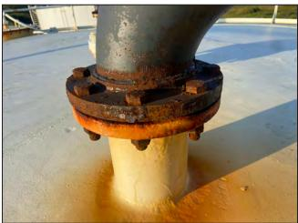
Photo 47: Detail view of gooseneck vent.
