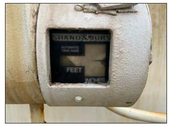
Photo 18: Detail view of autogauge readout.
