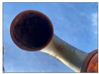
Photo 46: Detail view underneath gooseneck vent with no screen.
